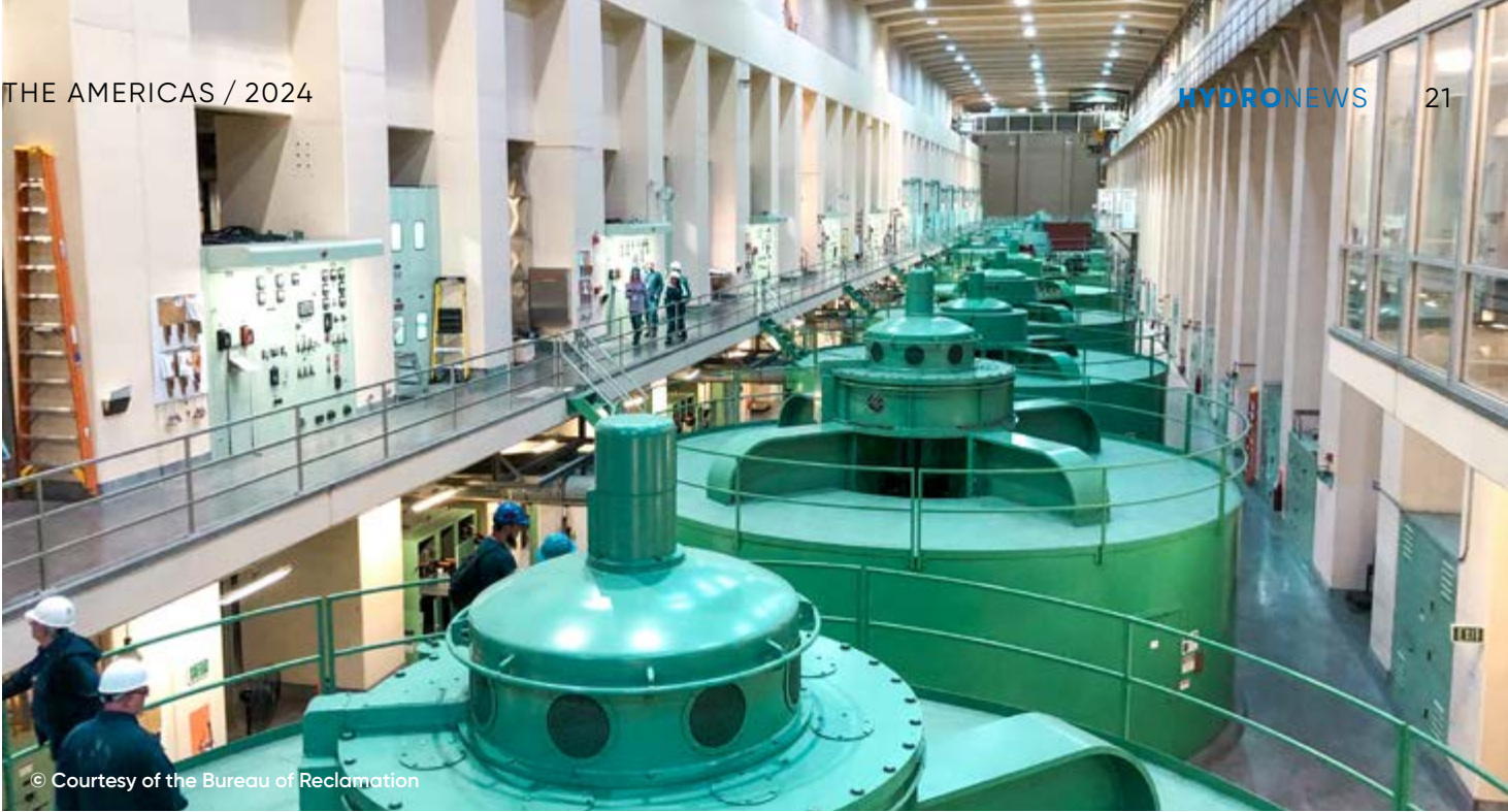
Unit hall of John W. Keys III pumped storage plant at Grand Coulee hydropower complex
