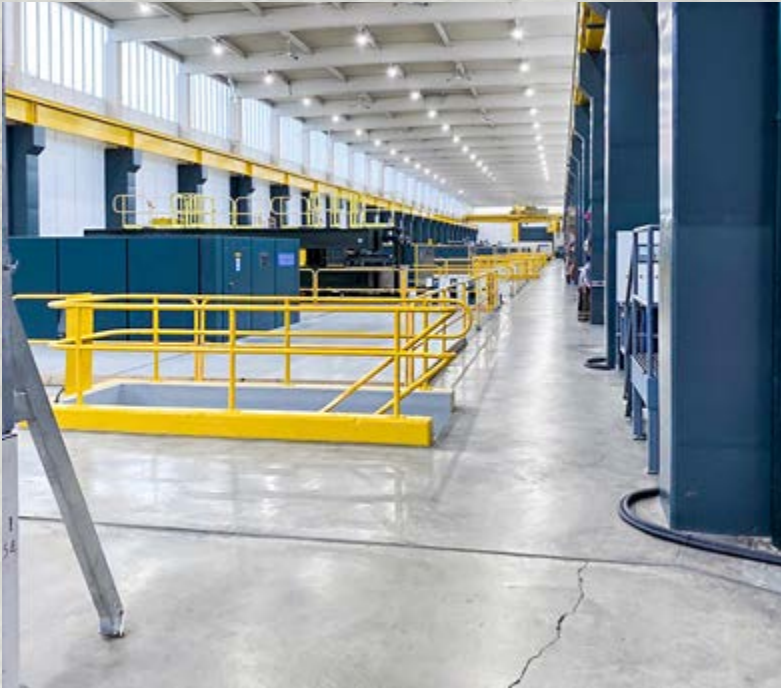
Good housekeeping practice – clear walkways and caution tape to delineate laydown
