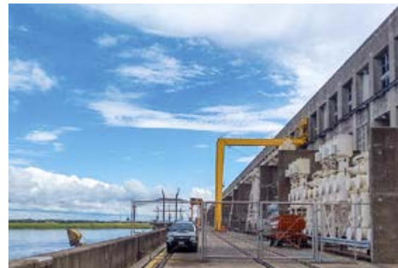
Yacyretá hydropower plant on the Paraná River, Brazil
