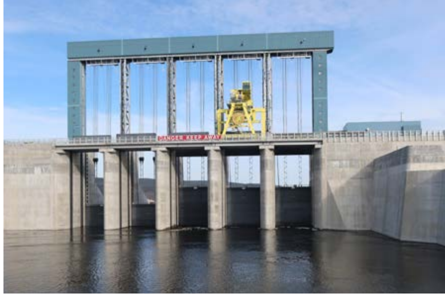
Gates at Muskrat Falls hydropower plant
