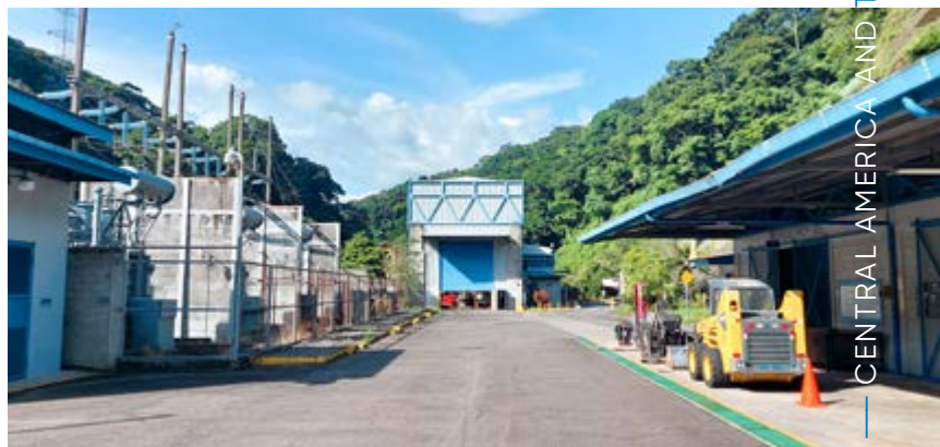
Powerhouse and substation of La Garita hydropower plant, Costa Rica
