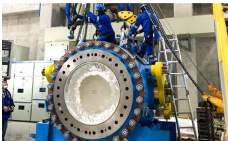
Installation of spherical valve at Huanza hydropower plant
