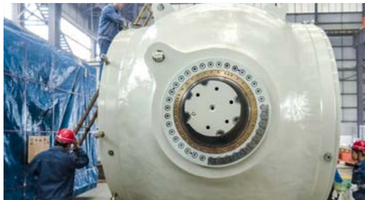
Inspection of main inlet valve, Coca Codo Sinclair hydropower plant
