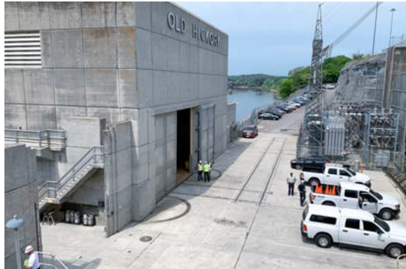
Powerhouse, Old Hickory hydropower station
