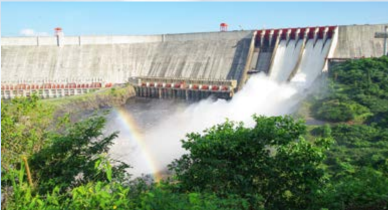
Simón Bolívar 'Guri' hydroelectric power plant
