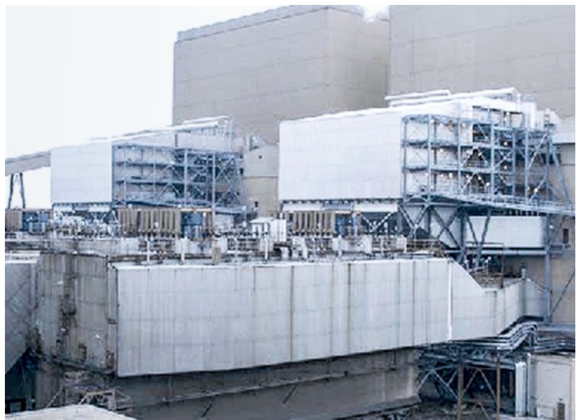
High-dust configuration at Hoosier Energy Merom Power Station, Units 1 & 2, Sullivan (IN), USA
