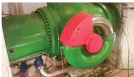
t Spherical valves after refurbishment
