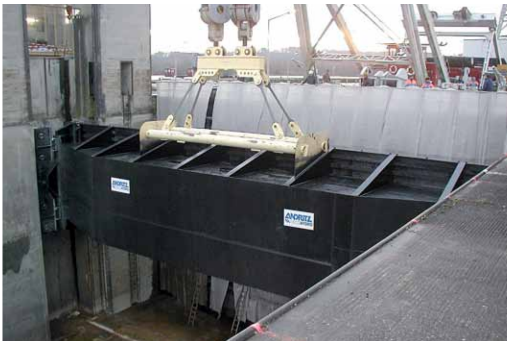
t Installation of double hook gate at HPP Wallsee Mitterkirchen, Austria
