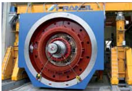
180 t heavy generator moved into machine-building using mobile rail track
