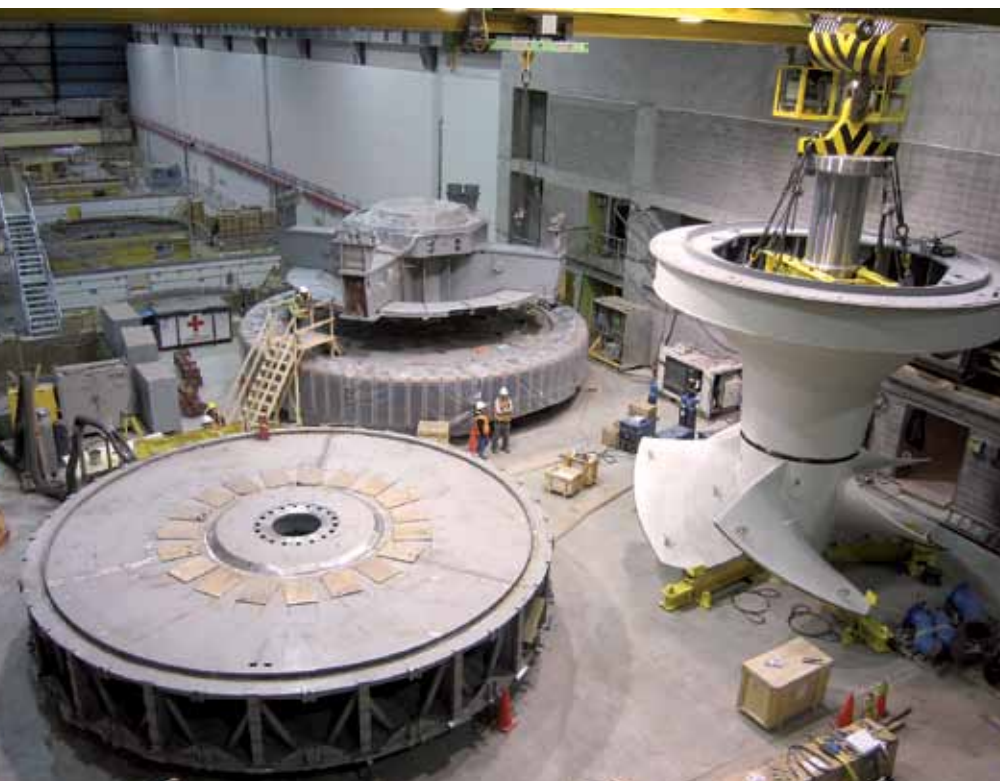
† Efficient use of assembly area by stacking of lower bracket on top of completed rotor
