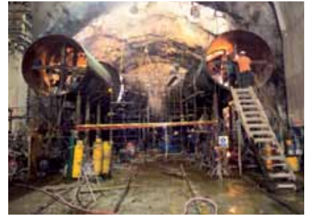
‡ Bifurcation site supervision erection
