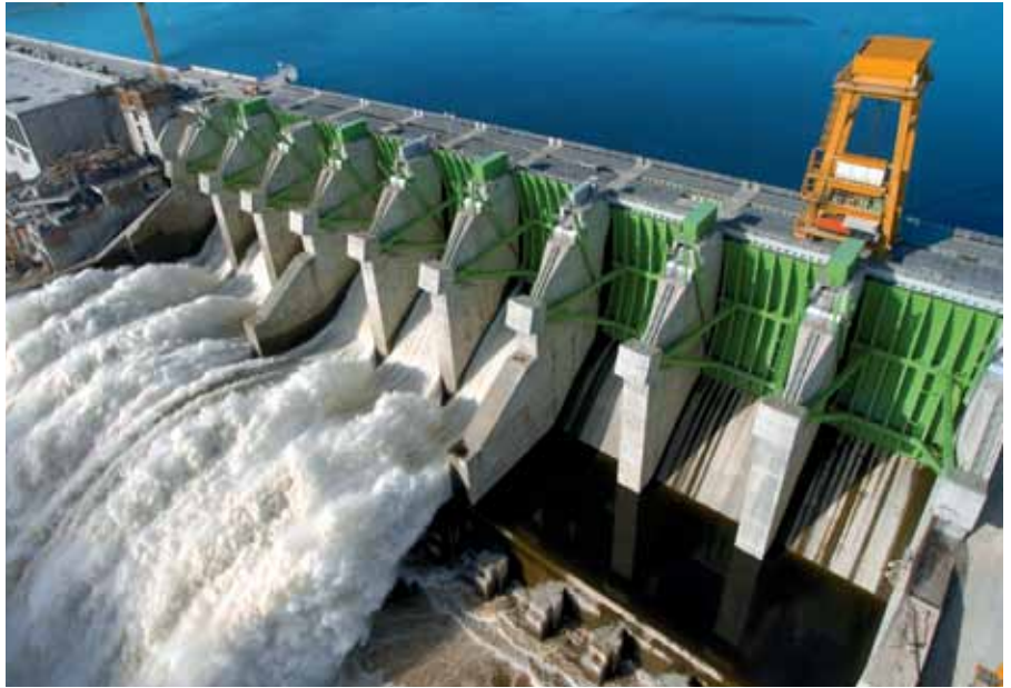
s Spillway gates at HPP Caruachi, Venezuela
