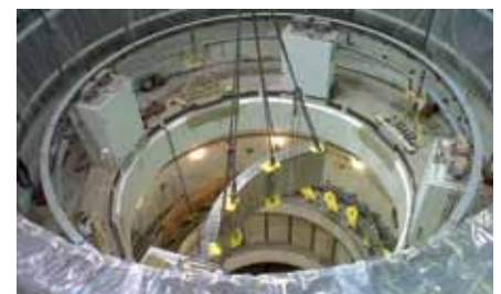
† Installation of discharge ring
