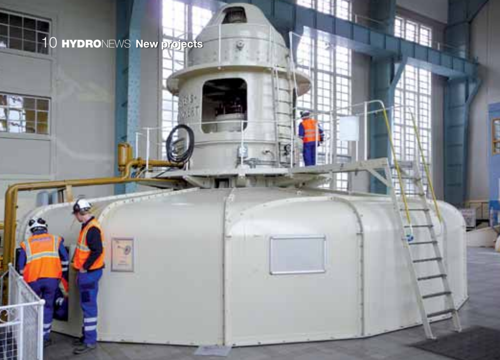
s Ardnacrusha during pre-design inspection
