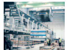
Lifting into the machine hall
