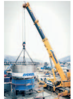
Two become one: on-site assembly at Pöls
