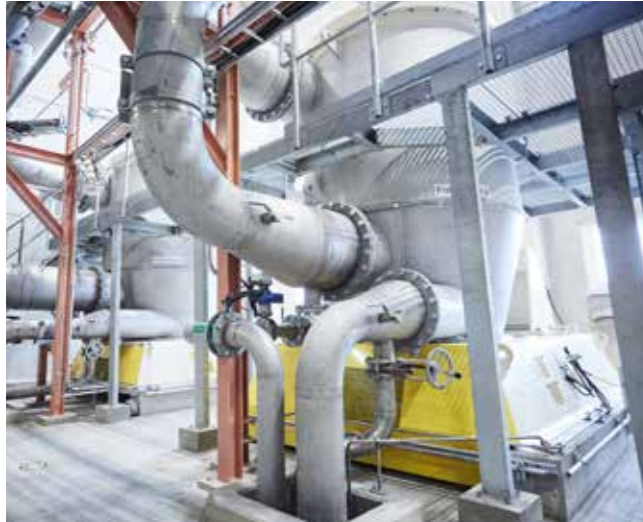
The fractionation section comprises a combination of existing equipment and a ModuScreen A with a matched screen basket/rotor concept.
