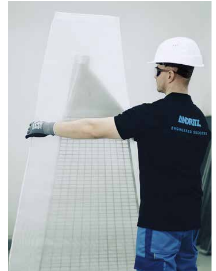
Installation of new filter bag
