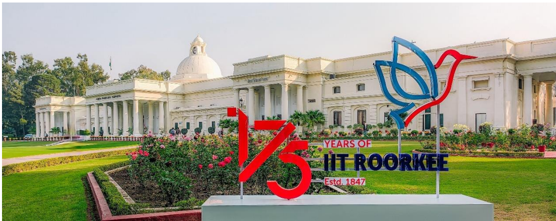
James Thomson Building, Indian Institute of Technology Roorkee
